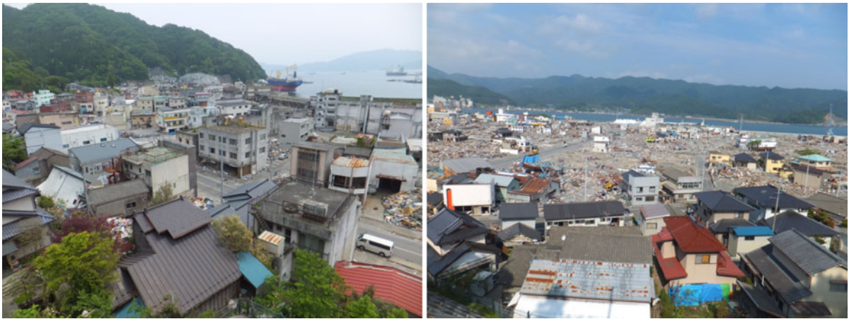
Figure 4 Damage from the tsunami inundation of Kamaishi city with a maximum runup height of 11.7 m (1/6/2011) and of Ofunato city with a maximum runup height of 10.9 m (1/6/2011)
