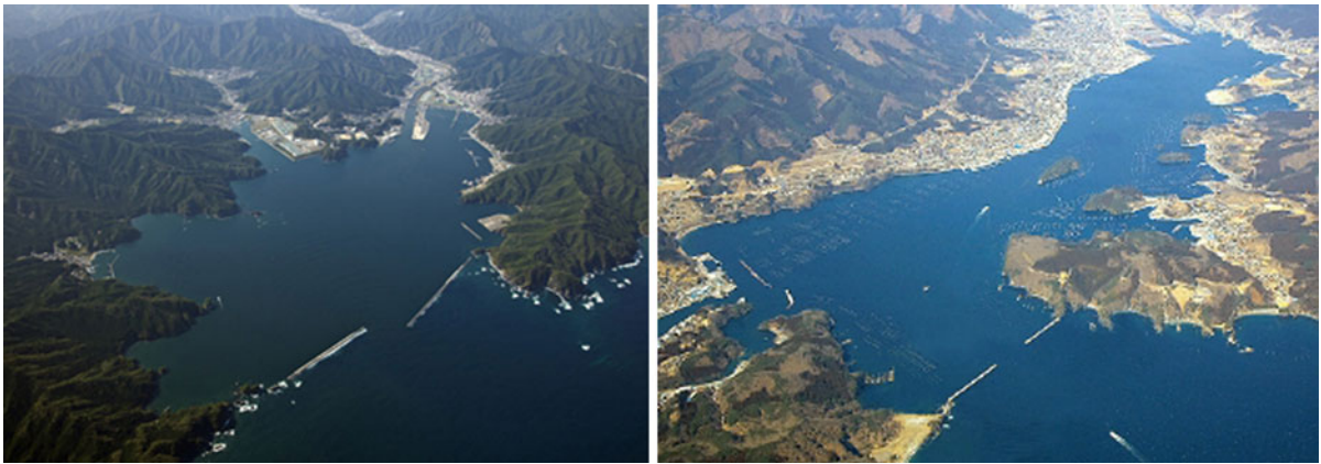
Figure 3 Tsunami breakwaters in Kamaishi city and in Ofunato city (before the 2011 tsunami)
