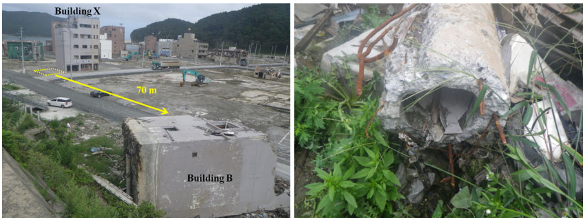
Figure 20 Building B, which was moved 70 m from its original location ( upper-left corner ), and a detailed picture of a pile foundation from building B (3/9/2011)
