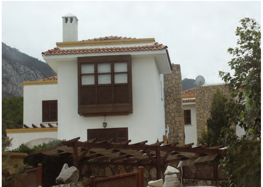
Figure 6. Some recent housing developments carrying traditional details of the past (F. Özersay).
