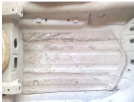
Fig. 4. Photographic image of surface damping treatment applied on the floor panel.
