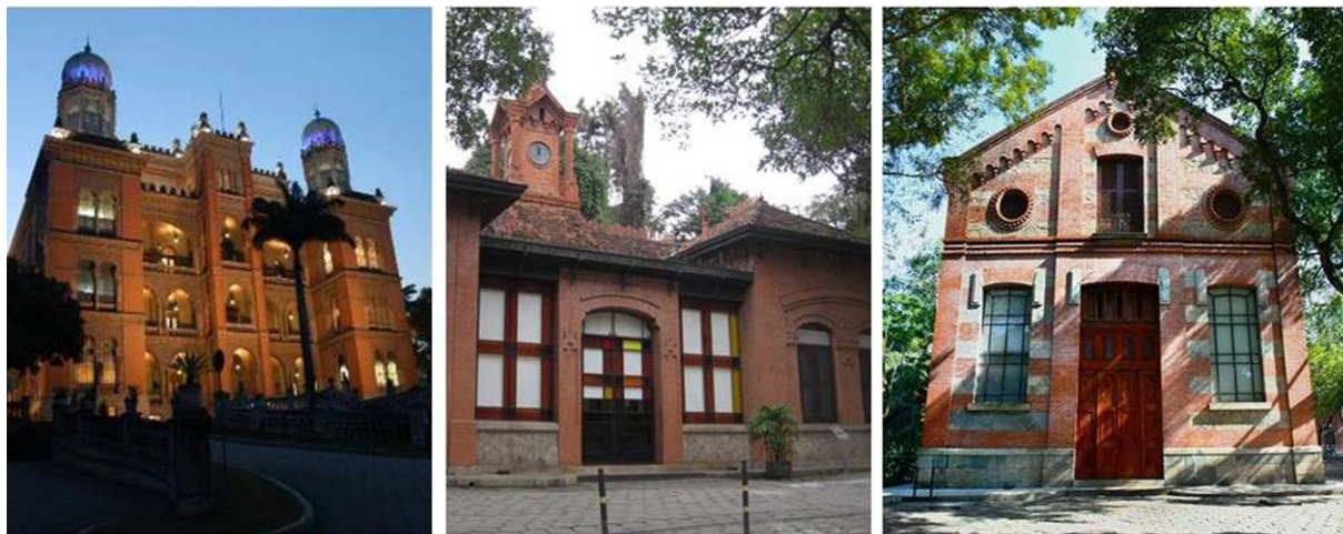
Figure 1 – Moorish Pavilion, Stable, and Clock Pavilion - Fiocruz's historical buildings. Source: Fiocruz
