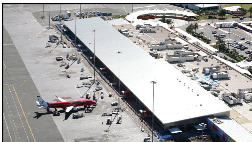
Figure 4.37: Redeveloped Gold Coast Airport Terminal – The First Purpose-built Low-Cost Carrier Terminal in Australia (Source: MPN Consulting (2018))
