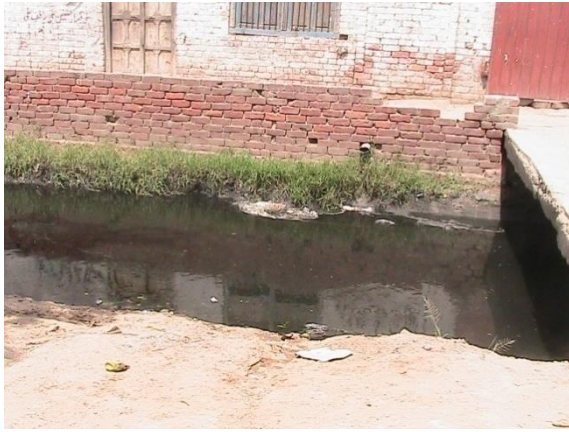
Domestic drain (PS-4), Site A
