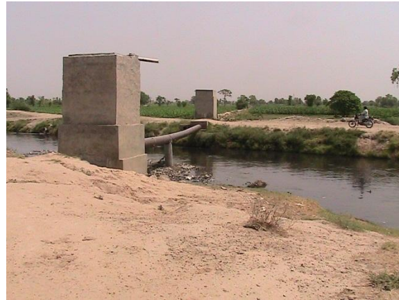
Paharang drain, Site B
