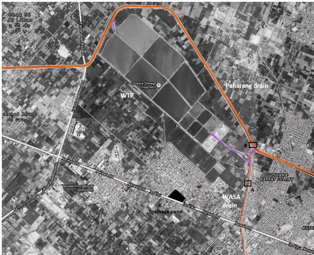
Figure 4.20: Location of the western site
