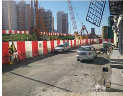
Fig. 5 - Commercial block around construction site in Taman Serdang Raya [19]
