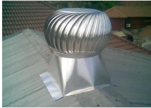
Fig. 1 - Roof ventilator mounted on the residential [8]
