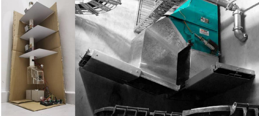
Fig. 2 - Prototype of waste chute system (left), and waste chute system by WasteTech Engineering [44] (right)
