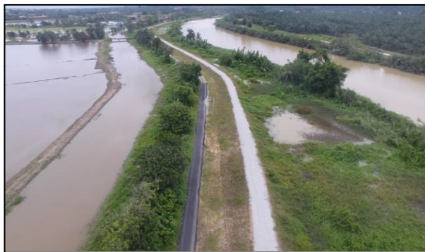
Fig. 2 - Sungai Kerian levee system
