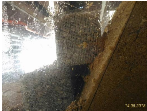
Fig. 7 - Wire meshes inserted with gravel.
