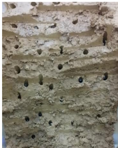
Fig. 14 - Infiltrating water hold in the burrow hole
