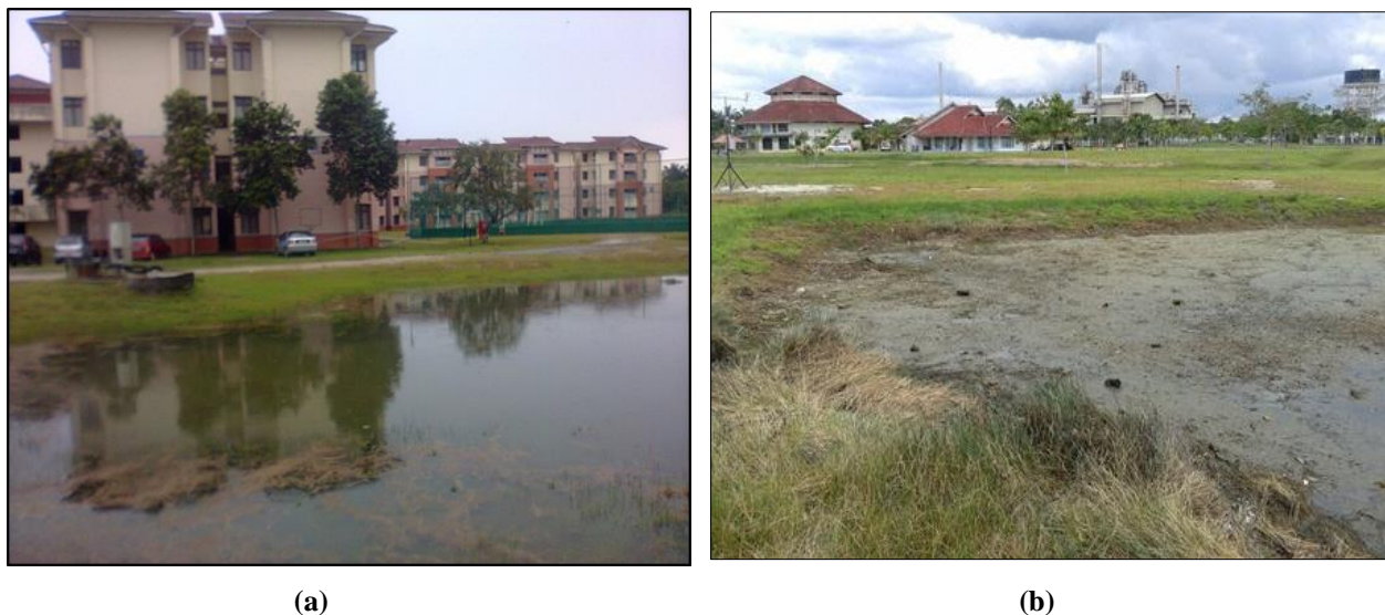
Fig. – (a) 1 RWH system in UTHM (b) dried pond after pumping
