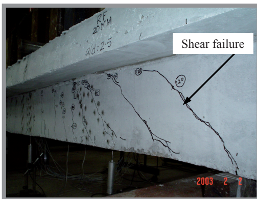
Fig. 2(a) Shear failure of control beam TT1a
