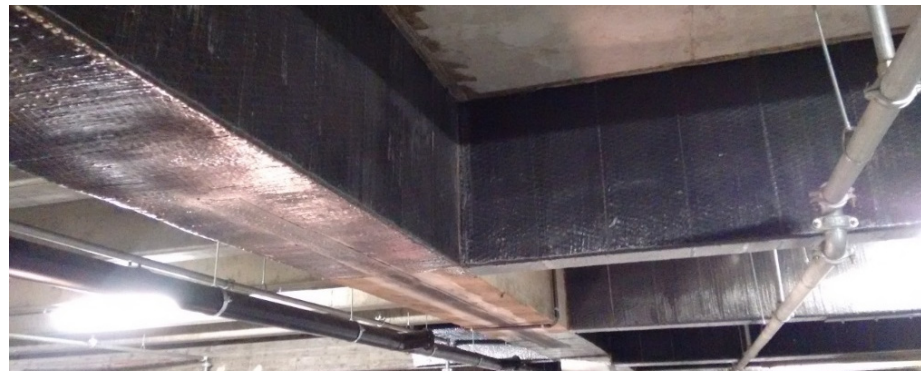
Figure 3. Example of FRP strengthening of beams in Ghent, Belgium.
