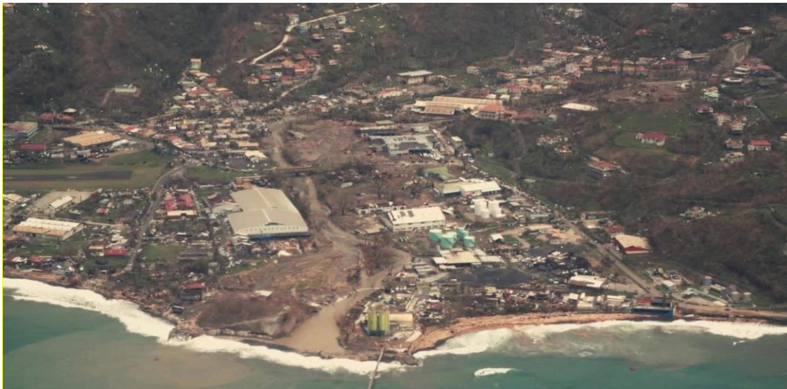
Figure 14. Dominican Coast Devastated Following Hurricane Maria (CNN, 2017).
