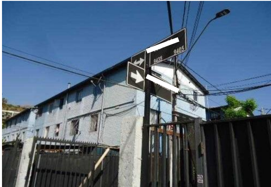
Figure 2: A building of houses, deprived area of Kupal
