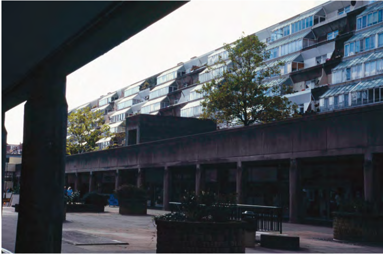
Figure 11.2 View looking due south of winter gardens to Foundling Court, prior to refurbishment
