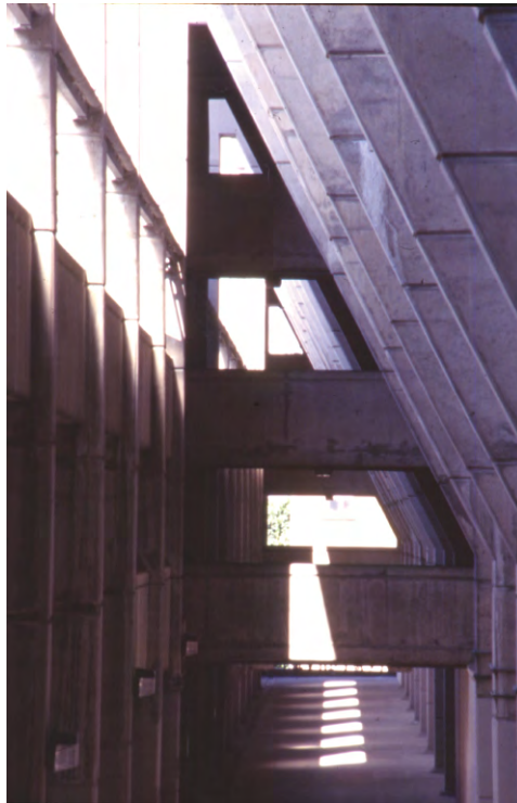
Figure 11.3 View through apex of concrete A-frame structure supporting housing block, with access level to atrium below
