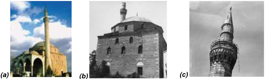
Figure 2.3: (a) View of Mustafa Pasha Mosque in Skopje; (b) & (c) Views of the damaged monument due to the 1963 earthquake (Krstevska et. al. , 2010)
