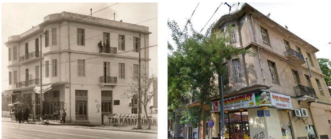
Figure 4a, 4b. Past and present condition of a case study. Photos: Koukou, T. 2016.
