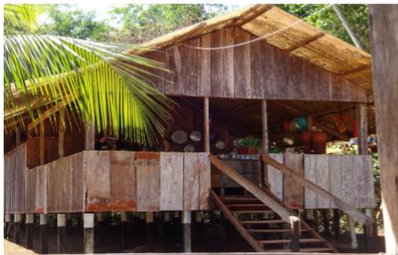
(a) Exterior of converted Brazil nut storage facility
