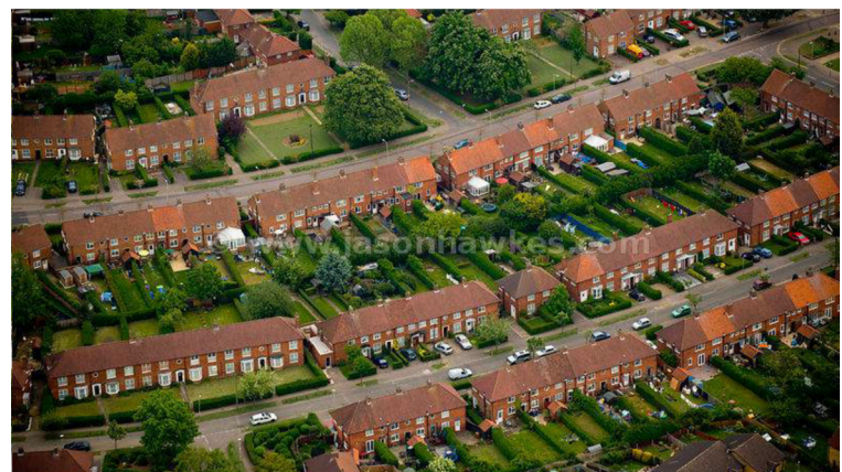
Letchworth Garden City, housing with a variety of green space types and sizes from setbacks to backyards to public squares
