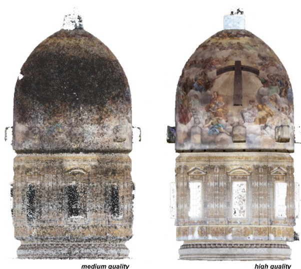
Figure 9. Image-based point cloud processed by the Parrot ANAFI dataset: detail of the dome obtained by the process in medium and high quality
