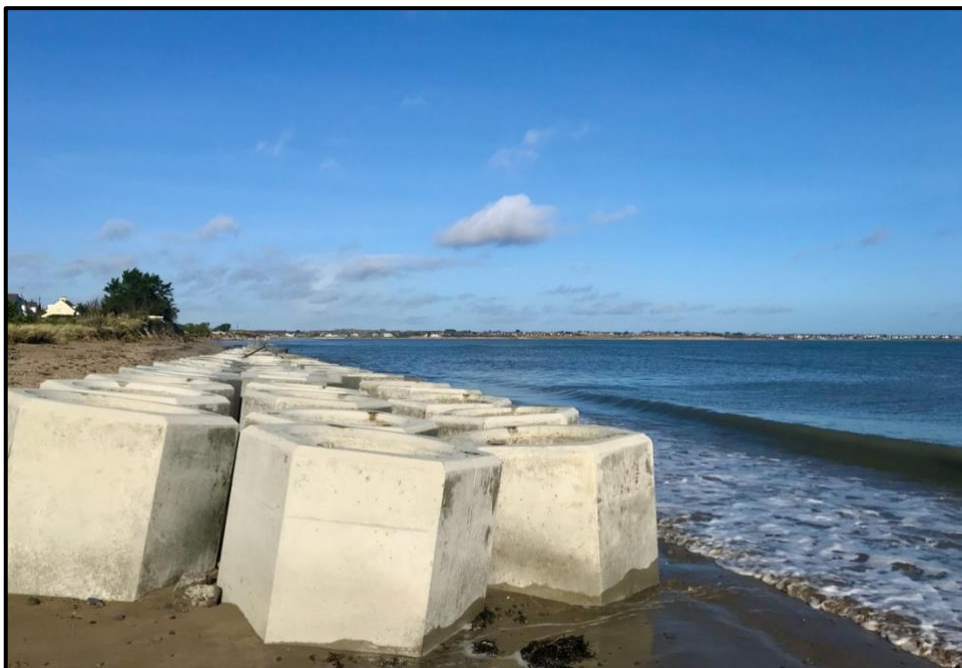
Figure 19: Seabees installed at the southern section of Burrow Beach.
