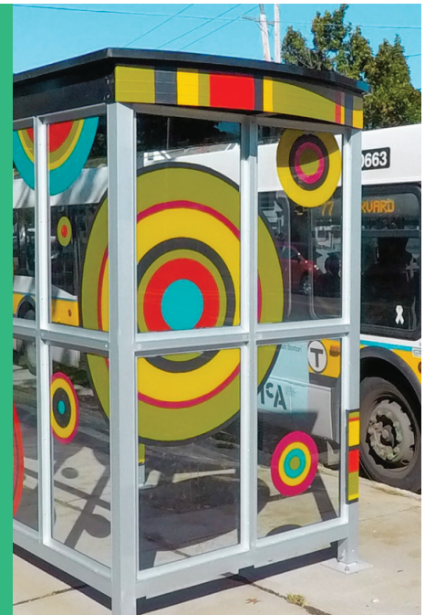
Arlington Bus Stop//Ad Hoc Industries
