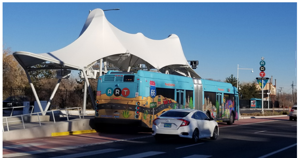
Figure 5: BRT stations can be aligned to the inside of the dedicated bus lanes (left), as in Albuquerque’s ART, or to the outside of the lanes (right), as in Richmond, Virginia’s Pulse BRT.
