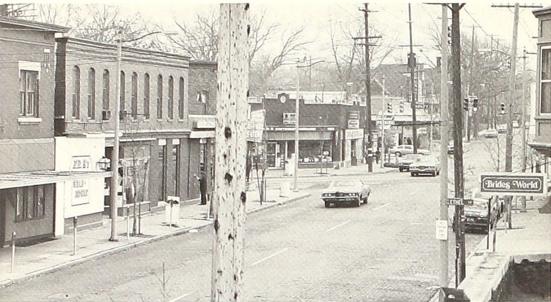
Wealthy-Lake Drive intersection, the commercial center of Easttown.
