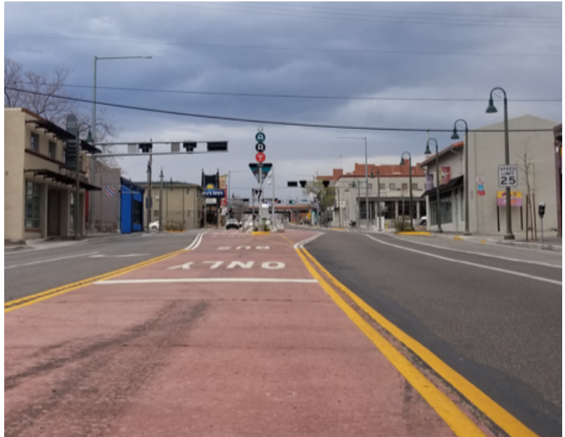
Bi-directional BRT lane in Albuquerque
