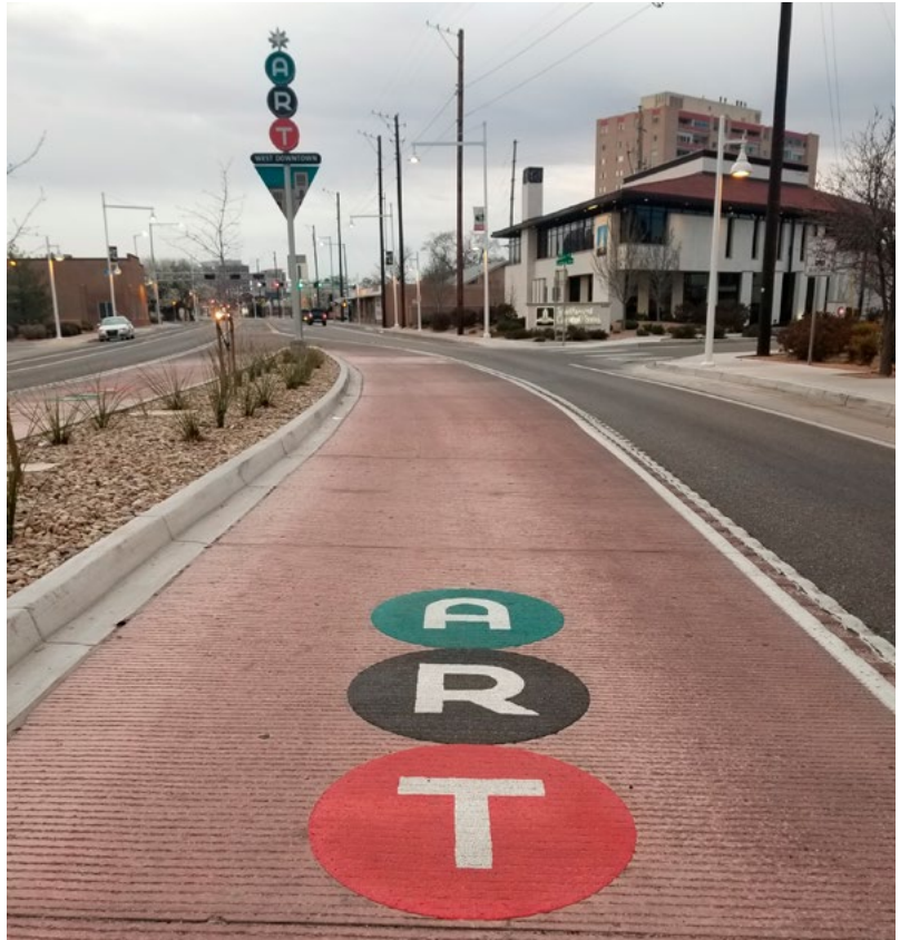
Figure 36: Just after West Downtown station the BRT lanes collapse into a bidirectional lane.
