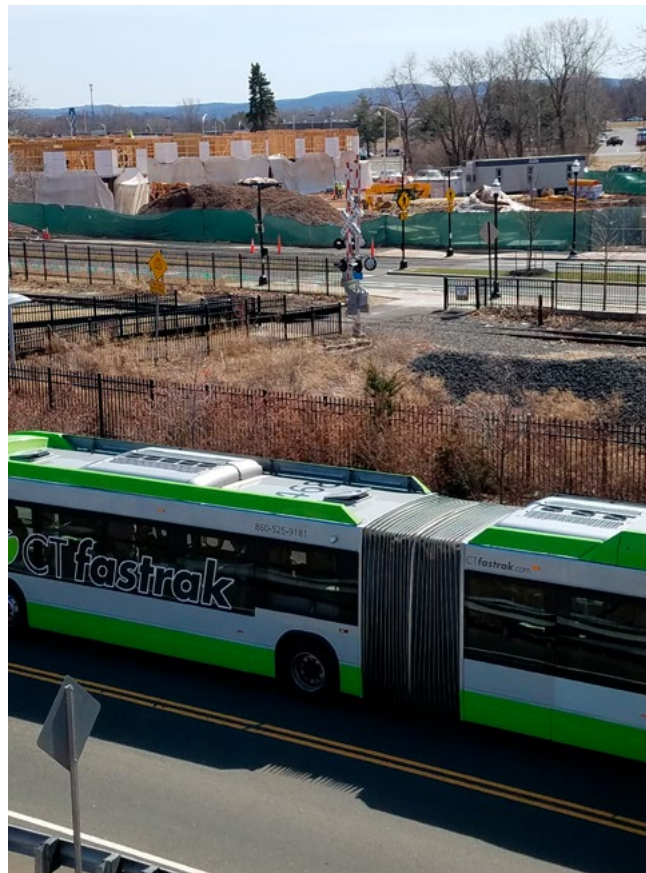
Figure 17: Construction of transit-oriented development, Columbus Commons, across from the CTfastrak station in New Britain
