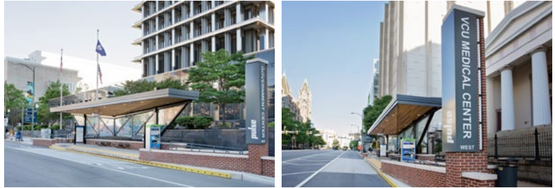
Figure 23: Curbside bus lanes and stations.
