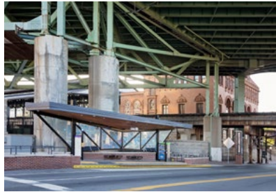
Figure 24: The brick and steel Pulse stations juxtaposed against diverse architecture.
