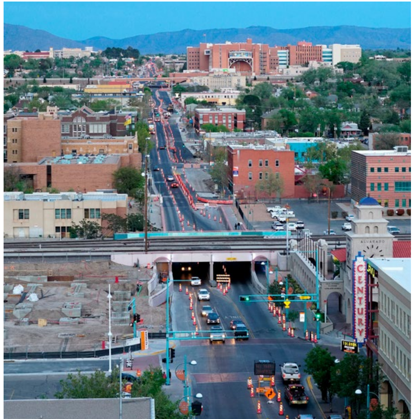
Figure 41: ART construction on Central Avenue east of downtown.
