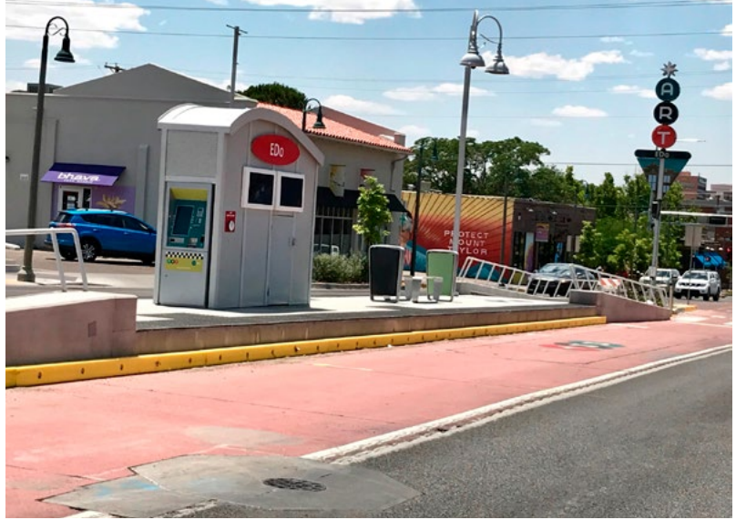
Figure 35: Median-aligned BRT lanes are colored red and separated from mixed traffic by a rumble strip.
