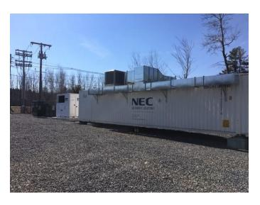
View of the battery storage unit at the Chocksett Road Substation. Shown is the battery container, labeled NEC; the 2 MW inverter, in a separate white container; and two transformers. Photo courtesy of SMLD.
