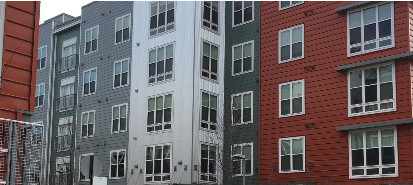
Everett Batch Yard, Massachusetts
