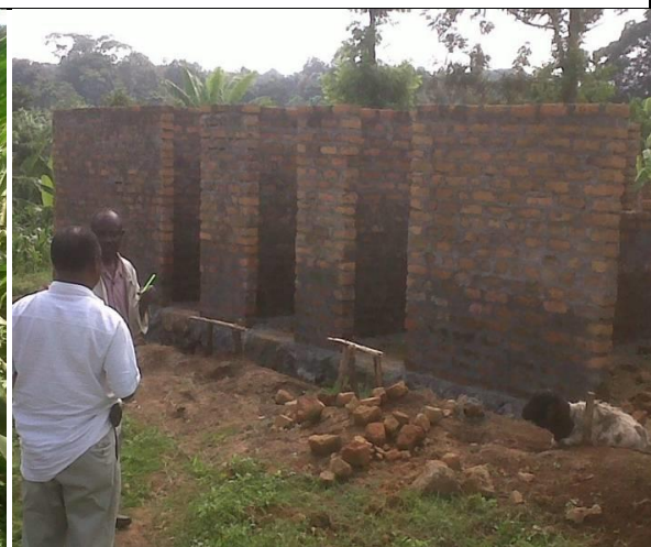
Figure 4.12: A Storage Facility under Construction, Kibosho Area
