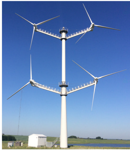
Fig. 2.4. Vestas multi-rotor wind turbine. Source: [35]
