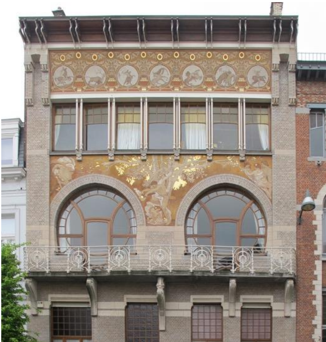
Fig. 22: Hotel Ciamberlani, Brussels (1897), by Paul Hankar and Albert Ciamberlani. Restored front elevation.
