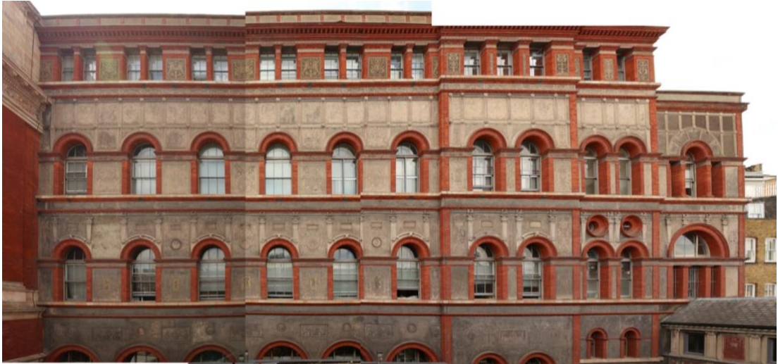
Fig. 28: Victoria and Albert Museum, London (1871 – 73), by F. W. Moody, F. E. Wormleighton, H. W. Foster, O. Gibbons, W. Wise. Composite elevation of the upper storeys of the Sir Henry Cole wing, formerly the Science Schools.
