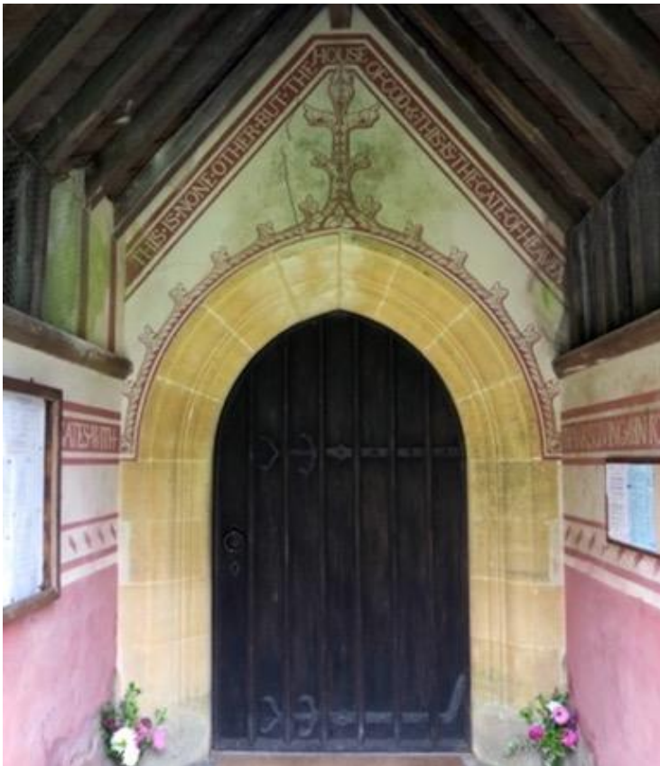
Fig. 43: St. Peter's Church, Hornblotton, Somerset (1873), by Sir Thomas Graham Jackson, architect, and F. E. Wormleighton and O. Gibbons, artists. South porch heralding the pink and white colour scheme of the interior, and the use of text on the walls.
