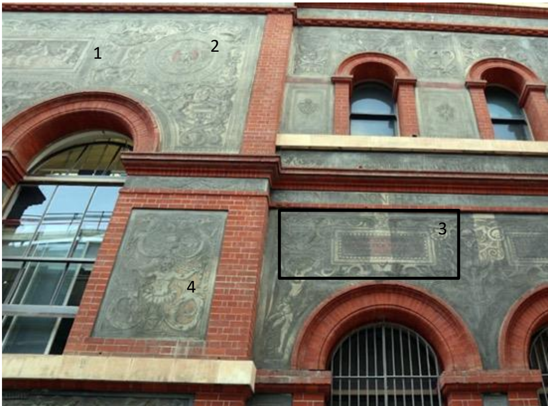
Fig. 31: Victoria and Albert Museum, London (1871 – 73), by F. W. Moody and his team. This is same part elevation as figure 30, showing classical scenes (1); roundel of contemporary notable figure (2); panel containing dedicatory text, ‘These experiments in plaster designed by F. W. Moody’ with the date ‘1872’ immediately to the left (3); and writhing classical decorative grotesques and surrounds (4).
