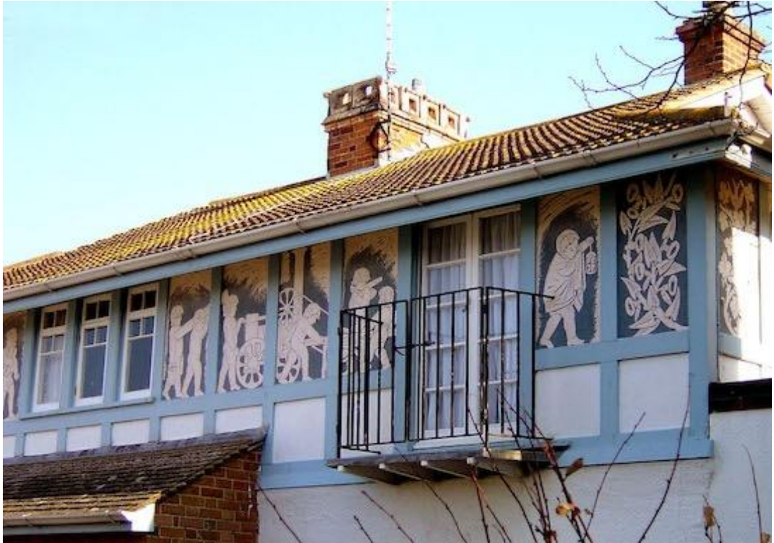
Fig. 59: 'Old coach House and Sunny Lodge', Birchington, Kent (1882), by John Pollard Seddon, architect, and George Frampton, artist. These panels are perhaps the most charming with the early locomotive and the hooded figure clutching a lantern; they have retained their character and the sketchy surround treatment visible in figure 57 despite later overpainting.
