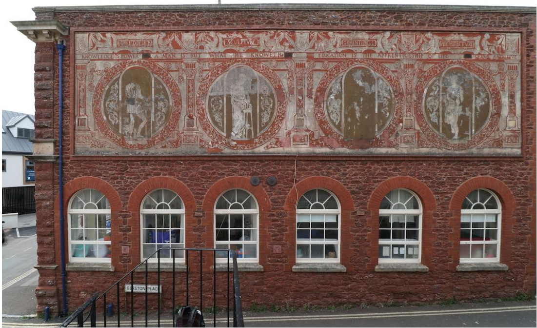
Fig. 10: Former Paignton Art College, Devon (probably completed 1908), by Arthur George Wallis. Sgraffito to gable.
