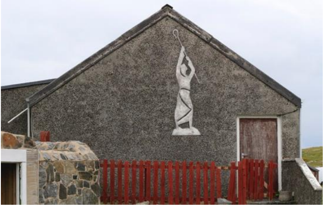
Fig. 17: Gable to hall adjacent to St Barr's Catholic Church, North Bay, Barra, Outer Hebrides (date unknown), artist unknown. The precise technique employed is uncertain but the figure has been created by cutting into the render surface.
