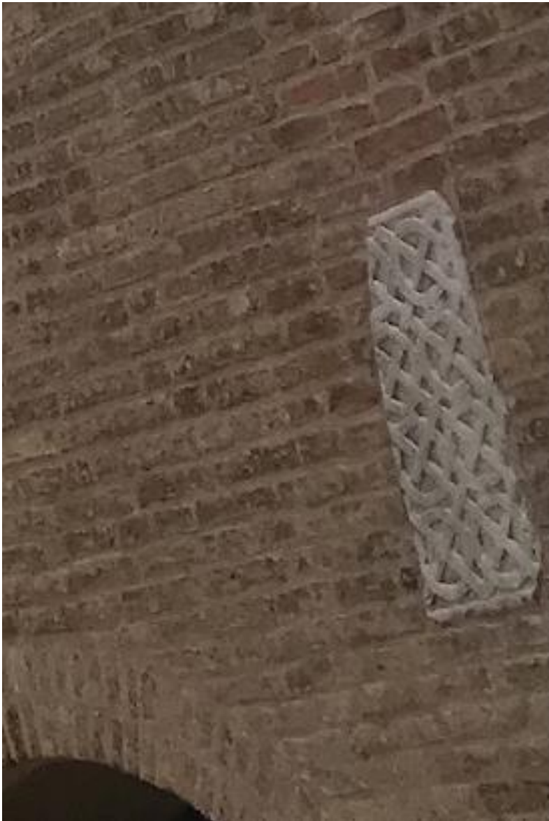
Figure 27: Cloister of the church of Santo Stefano, Bologna, Italy (2021). This surviving detail appears to match that shown in the 1875 engraving in figure 26. It appears quite crude suggesting it is either applied stucco detail or very early sgraffito. It has similarities to Moorish work in medieval and early Renaissance Spain
