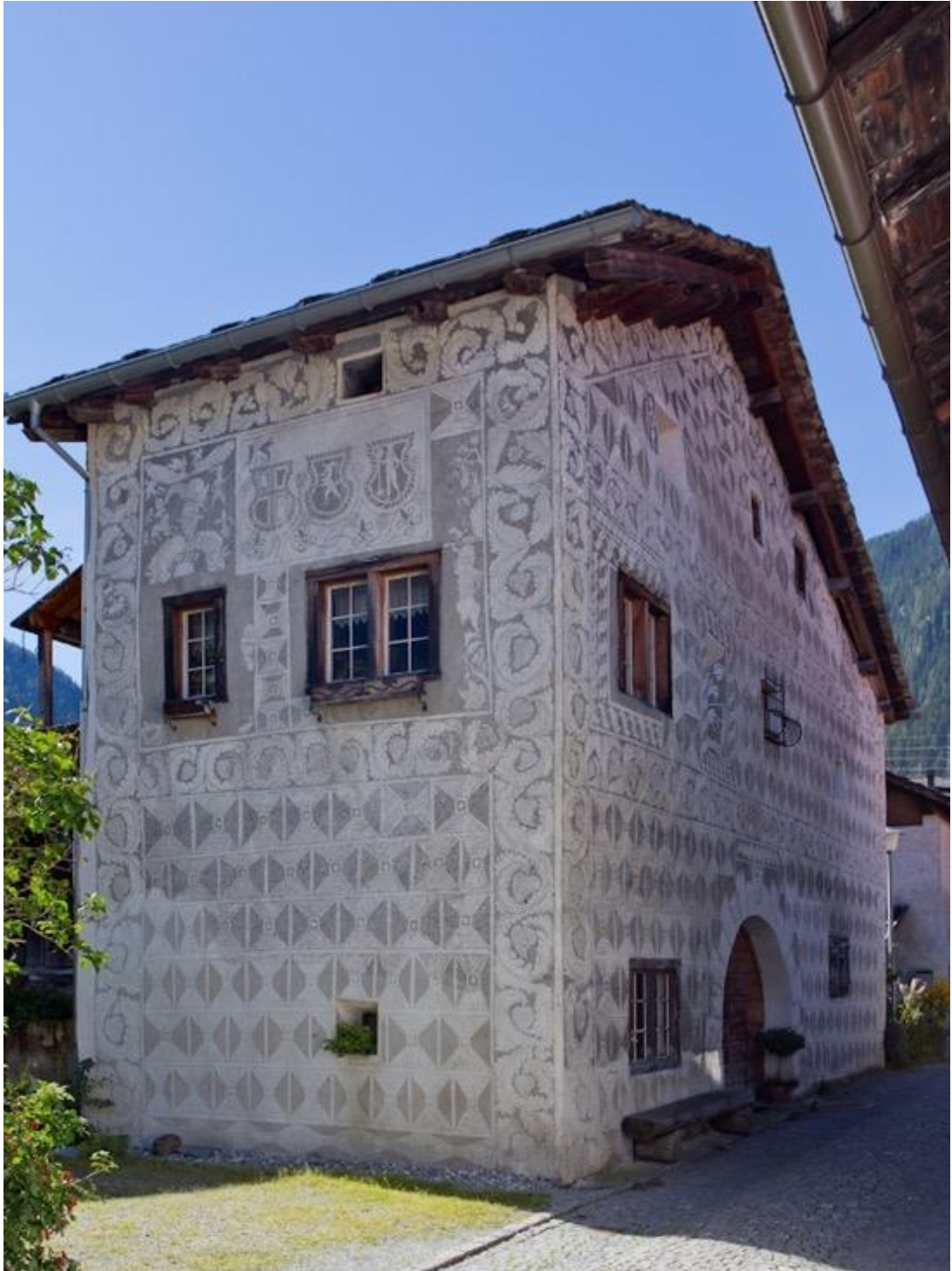
Fig. 13: Padrun House, Andeer, Switzerland (1501). ‘...flamboyantly unrelated to the structure of the building...,’ although not entirely so. Close inspection shows one band of circular pattern marking edges and floor levels and framing a second lozenge one; but the effect is dazzling.
