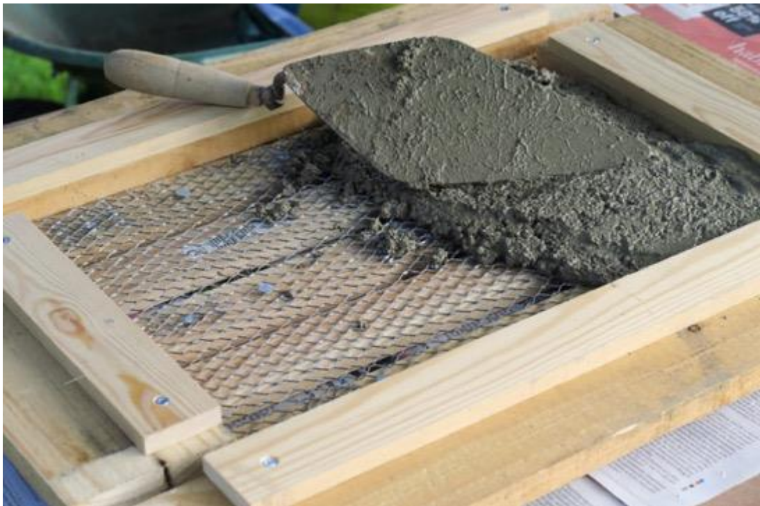
Fig. 5: Test panel 1. Application of cement sand base coat.
