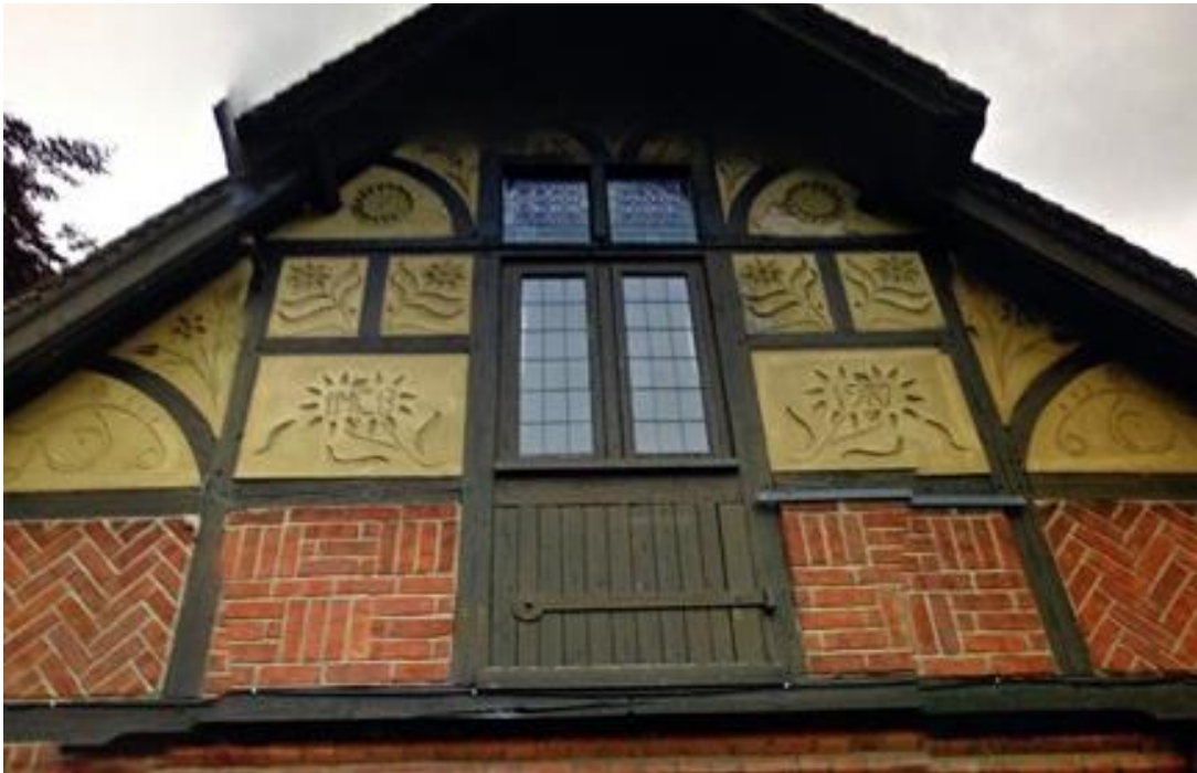
Fig. 52: 11 Castle Street, Buckingham (c1875), by Edward Swinfen Harris. A rustic character created by the construction as well as the rather crude, apparently stenciled, sgraffito.
