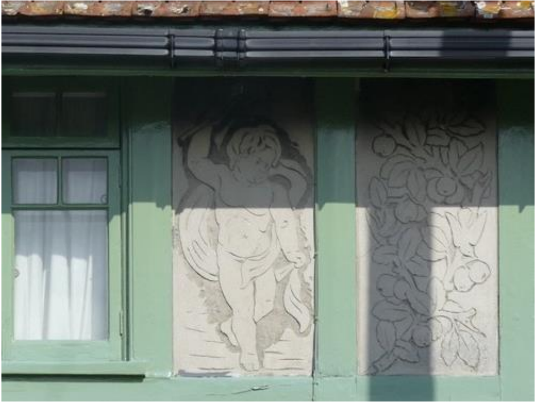
Fig. 57: 'Poets' Block', Birchington, Kent (1882), by John Pollard Seddon, architect, and George Frampton, artist. Weathered but apparently original finish. Note the execution of the figure and the foliage with a bird compared with those in figure 58.
