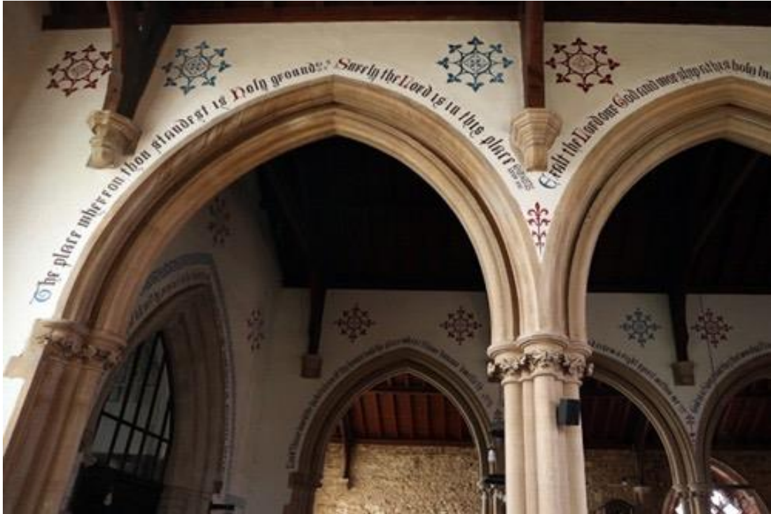
Fig. 25: St Mary the Virgin, Maulden (c1859), by Benjamin Ferrey. South aisle and nave sgraffito.
