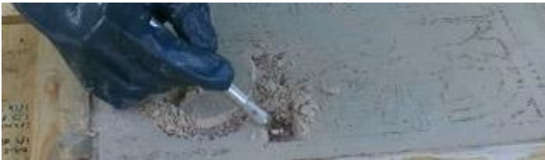
Fig. 16: Test panel 1. Starting to clean off the residual plaster on the colour surface.
