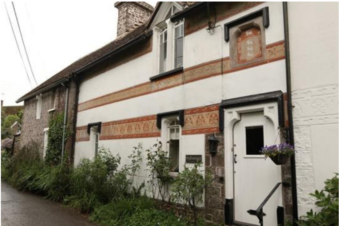
Fig. 61: Cottages, Down St Mary, Devon (c1875), attributed to Radford. A striking effect with modest means. Sgraffito on the right-hand property has been obliterated at upper levels and painted out at lower.
