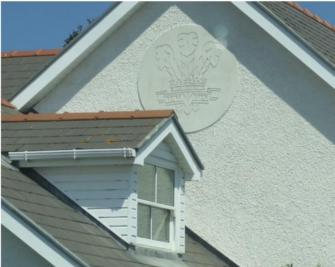
Fig. 18: South gable to house on main coast road south of Aberaeron, Ceredigion, Wales (date unknown), artist unknown. The north gable has an identical panel. This appears to be single coat sgraffito.
