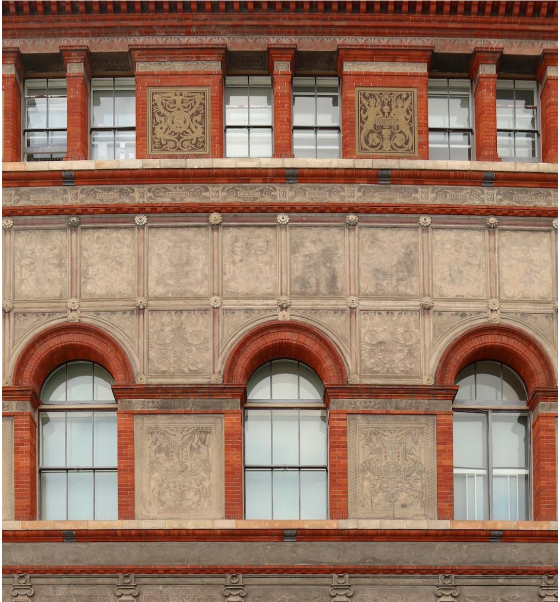
Fig. 29: Victoria and Albert Museum, London (1871 – 73), by F. W. Moody and his team. Detail of upper level with restored panels, showing grotesque designs with virtues listed in panels in a line beneath.
