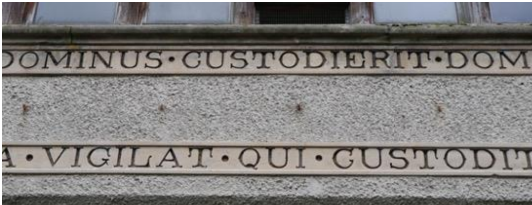
Fig. 28: Doveleys, Staffordshire (probably 1856), artist unknown. Detail of incised plasterwork on west elevation. The underlying render can be seen through the letters.
