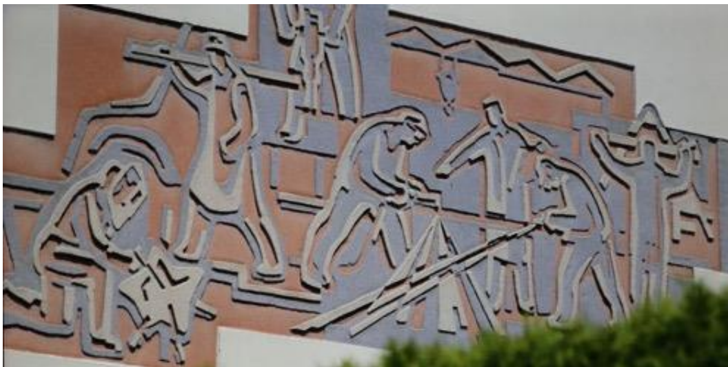
Fig. 27: Nürnberg sgraffito (date unknown), artist unknown. Scene of construction workers. The depth of sgraffito using 'Putzschnitt' is easy to see.
