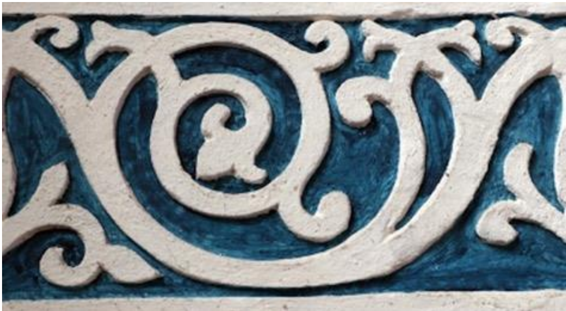
Fig. 26: St Mary the Virgin, Maulden, Bedfordshire (c1859), by Benjamin Ferrey. Dado detail showing infill repainting. This appears to have been carried out using Ferrey's patented stamped sgraffito method.
