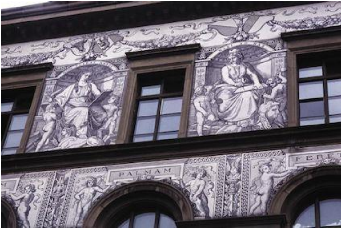
Fig. 16: Polytechnikum, Zürich, Switzerland (1858 – 1863), by Gottfried Semper, This shows the didactic and pictorial effect of Semper's sgraffito.
