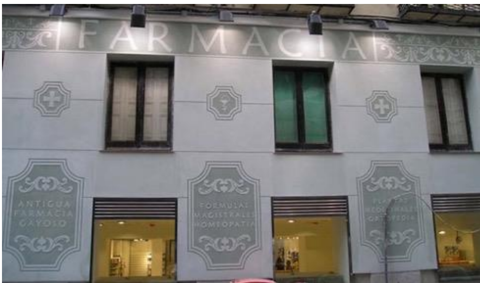
Fig. 16: The finished shop front.
