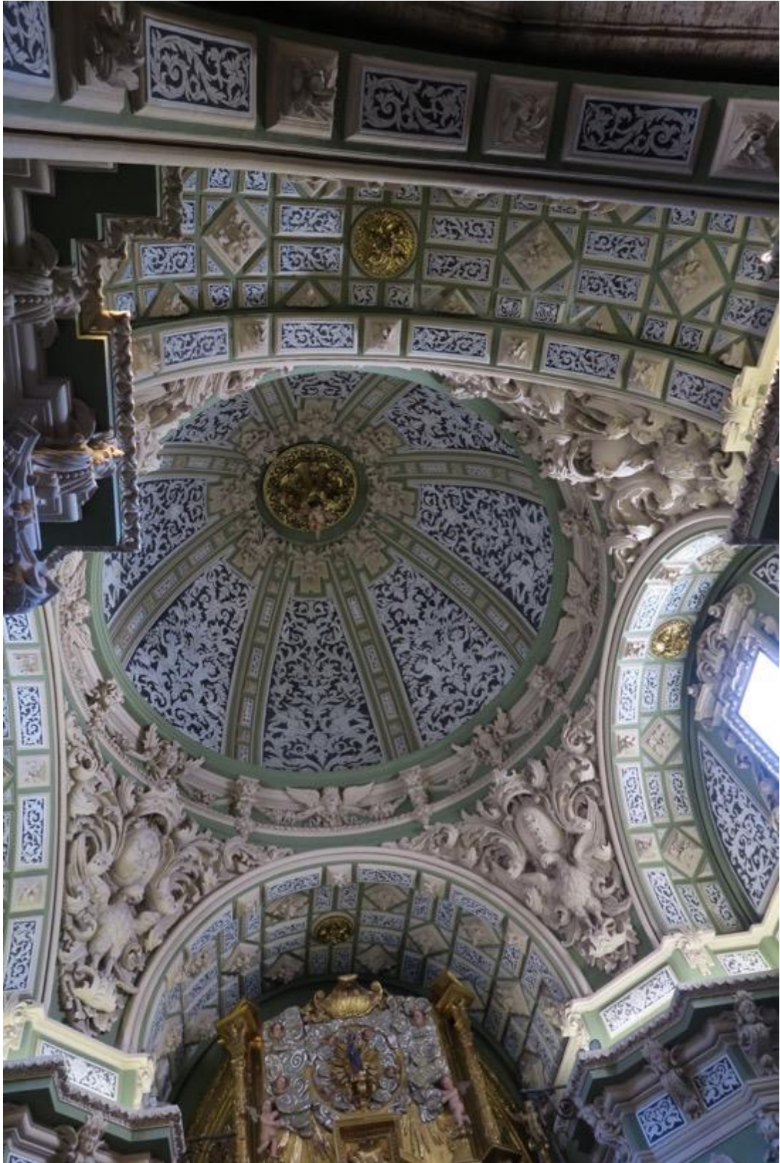
Fig. 15: Chapel of Santa Barbara in the Church of San Juan del Hospital, Valencia (from around 1700). Sgraffito on dome, arch soffits and wall panels.
