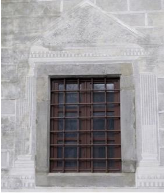
Fig. 5: Palazzo Lapi, Florence, Italy (after 1452). The impression of stonework created in sgraffito.
