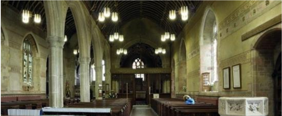
Fig. 33: Church of All Saints, Winkleigh, Devon (1871 – 72), by R. D. Gould and W. T. A. Radford. Nave looking east showing horizontal sgraffito bands.
