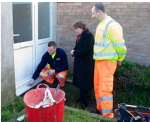
Figure 3: Installing flood doors, Liverpool
