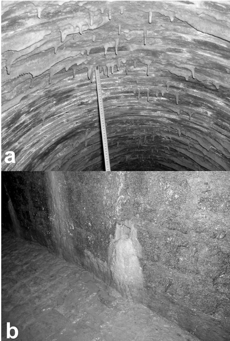
Fig. 6 - (a) Stalactites and draperies on the vault of the canal. (b) Flowstones on the walls of the canal (bricks are 30x20 cm).
