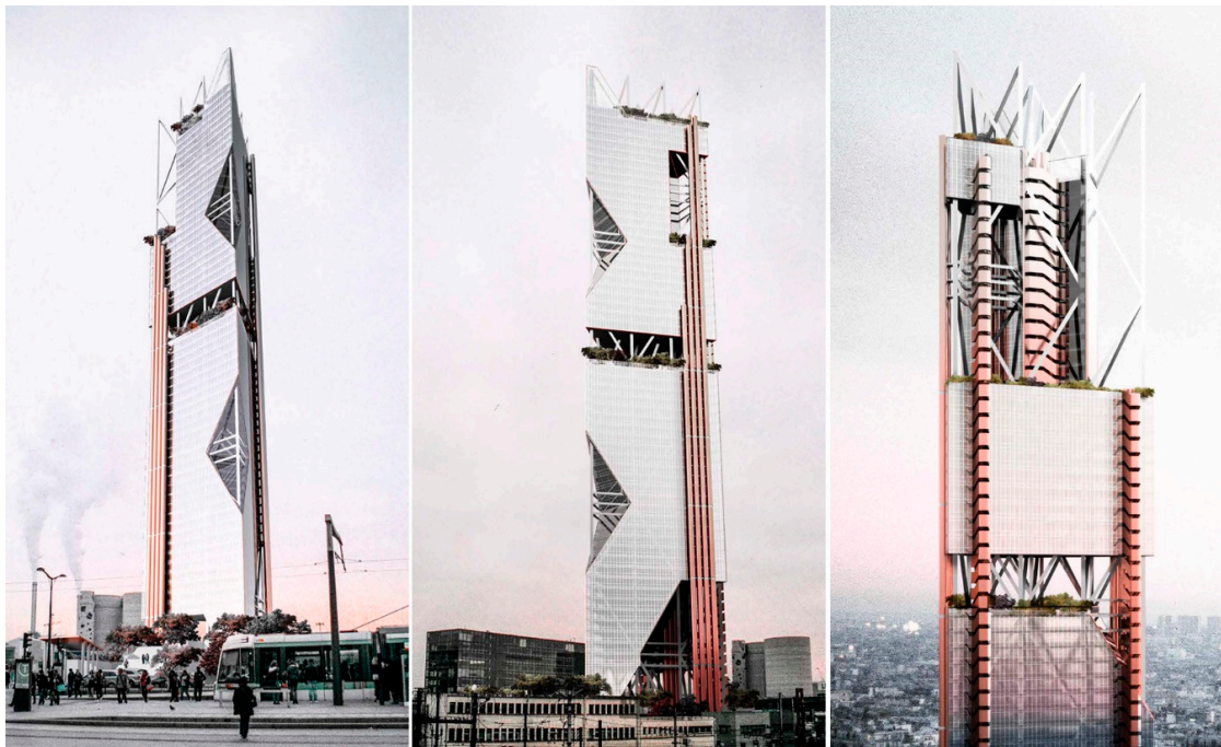
Figure 1. Rendering views of an applicative example of the tetrahedral structural system in the design of a tall building.
