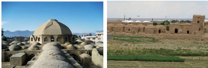
FIGURE 14-15 The effect of dome-like roof on skyline, Photo: Left: Laar city ©www.kojaro.com Right: Hossein- Abad-Kavir in Isfahan province ©Mahnaz Sarlak
