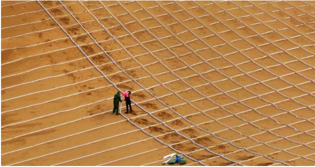
FIGURE 3 The use of degradable material by sand barrier technology (@europe.chinadaily.com.cn)
