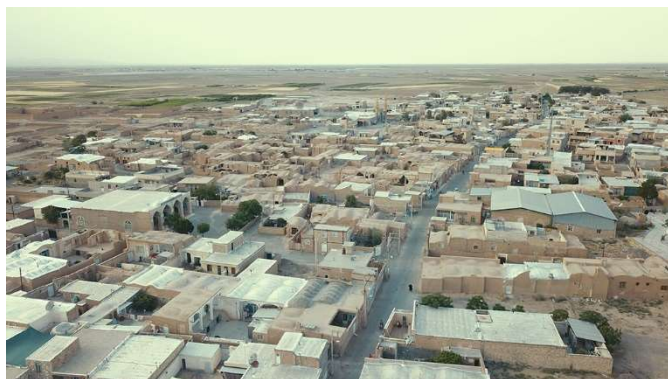
FIGURE 22 Urbanizzazione in TaherAbad village Photo by Mahnaz Sarлак using an unmanned aerial vehicle- 2019
