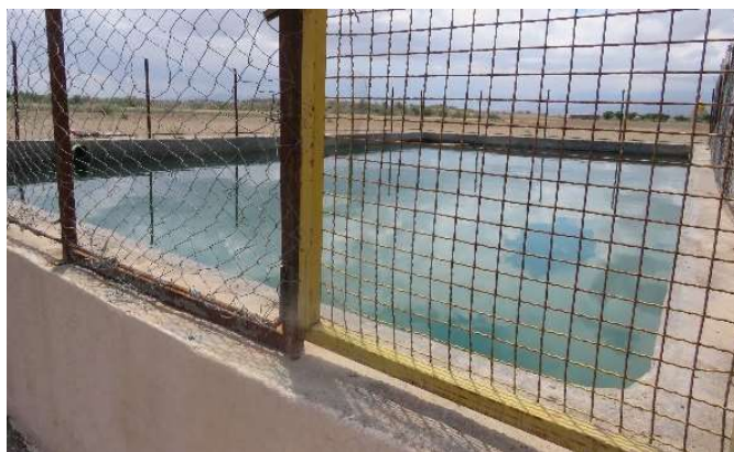
FIGURE 12 Pool with a capacity of 500 cubic meters in Ghasem-Abad village (photo by Mahanz Sarlak-2018)
