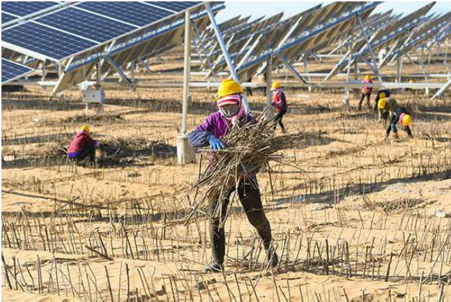
FIGURE 5 worker paves sand barriers between photovoltaic panels to prevent soil erosion at a photovoltaic power station of Kubuqi Desert (@xinhuanet.com)
