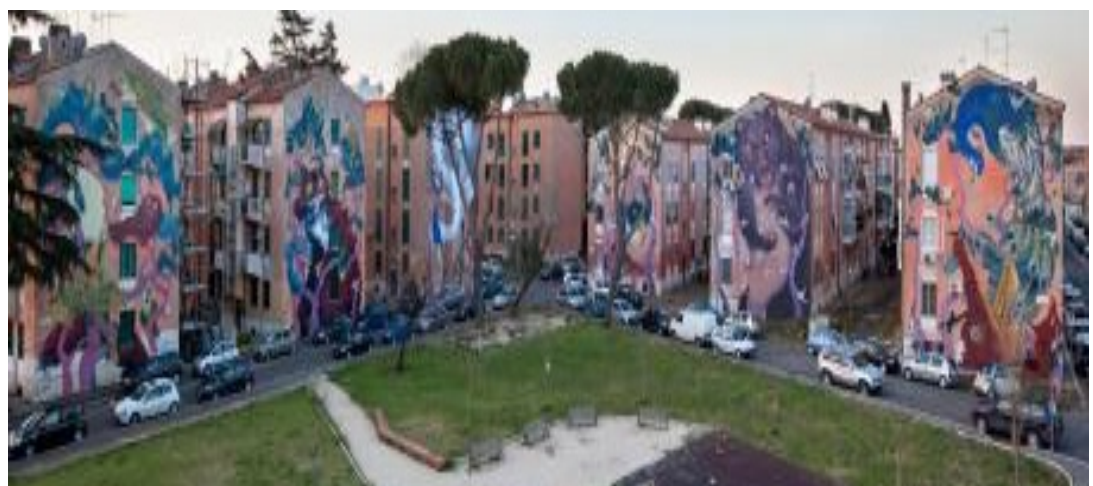
Figure 2- 18. Hitnes Murales on Tormarancia Ater houses, Rome. Photo by Muscella, V. (2015)
