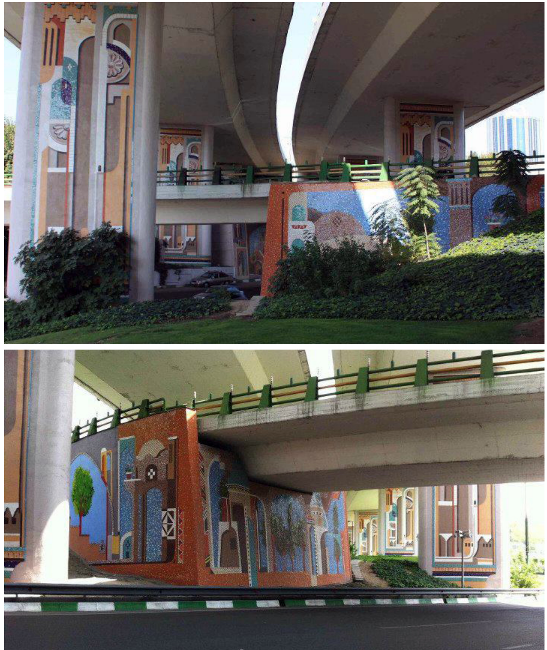
Figure 3- 8. Modarres Highway-Hemmat intersection, Fajr bridges. Photo by Mobasheri, S. (2018)
