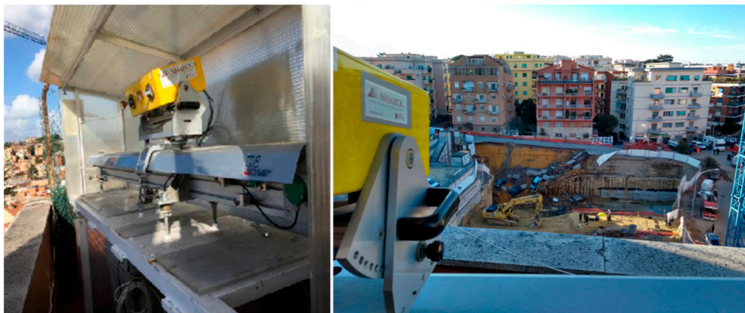
Figure 5. Terrestrial Synthetic Aperture Radar Interferometer (TInSAR) equipment deployed on the rooftop of a building located near the construction site.
