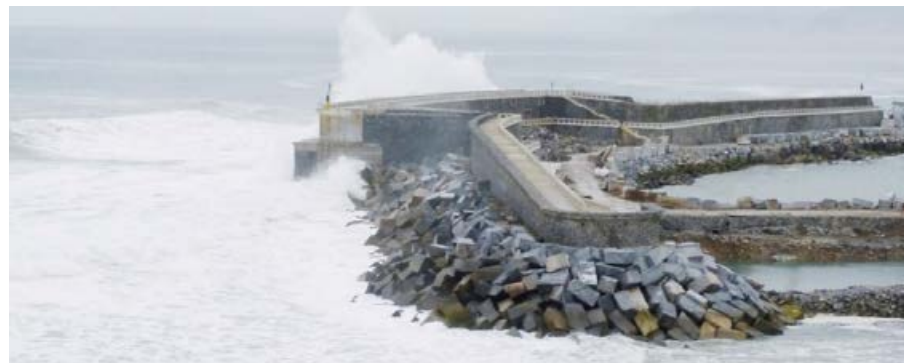
Figure 12. OWC plant installed in the bay of Mutriku (Spain) [54].
