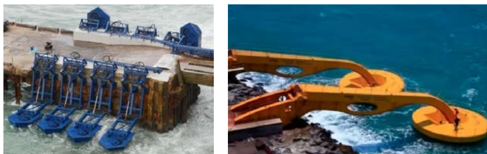
Figure 28. View of Eco Wave Systems installed on Gibraltar (left) [93] and Seahorse power take-off system (right) [94].
