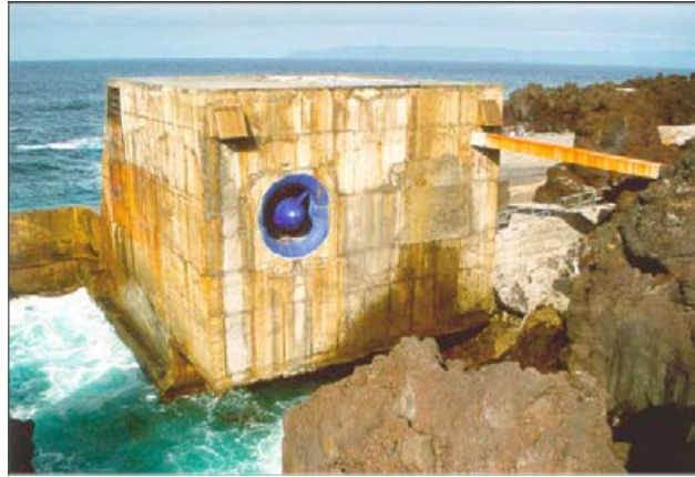
Figure 11. Back view of the OWC plant installed on the island of Pico (Azores, Portugal) (Reproduced with permission 5139250512092 from [50], Elsevier, 2016).
