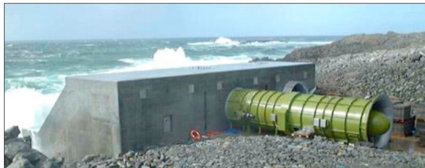
Figure 10. LIMPET OWC plant installed on the island of Islay (Scotland, UK) (Reproduced with permission 5139250512092 from [50], Elsevier, 2016).
