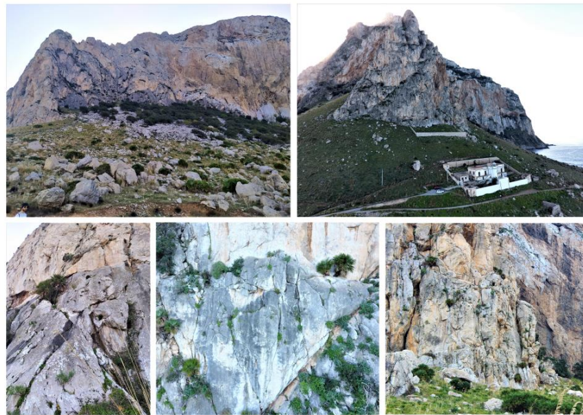
Figure 3. Discontinuities, unstable rock blocks, and boulders in the rock walls affected by rockfall phenomena.
