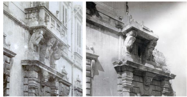
Figure 13. The balcony before and after the earthquake.
