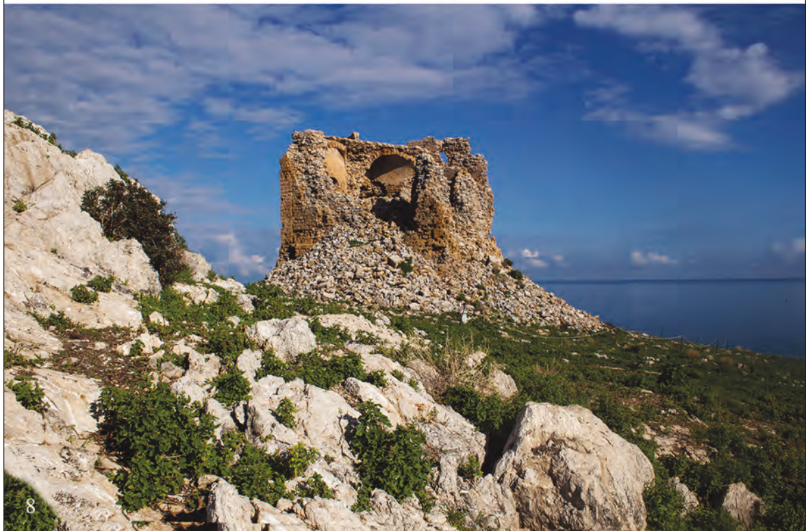
Figure 7. Isola delle Femmine, southern slope and the Torre di Fuori in the highest part of the territory.
