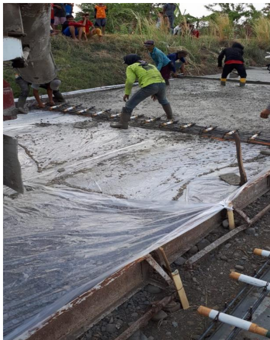
Gambar 4. Proses Pengecoran Beton
