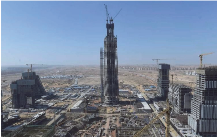
Figure 9. Iconic tower—Egypt’s new administrative capital.
