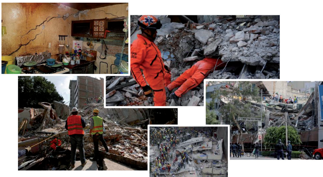
Figure 3. The Mexican earthquake from the 19 September 2017 led to significant building damage in the capital Mexico City and the states of Morelos and Puebla. The damage data in houses/buildings and soils characteristics highlights the correlation between damage drivers that little has been studied or they have not been fully understood.
