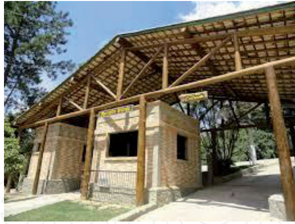
Figure 1. Treated wooden posts. Source: https://images.app.goo.gl/3eKubCdjmWMQdV2z6 .
