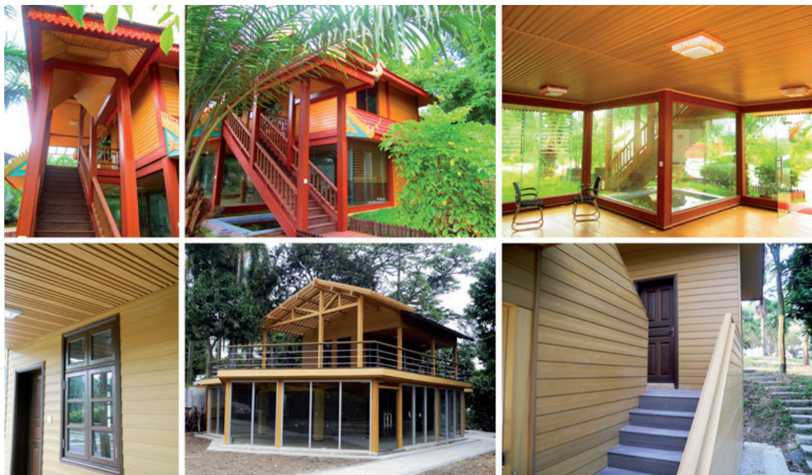
Figure 2. The applications of WPC in the indoor or outdoor ceilings and sidings.
