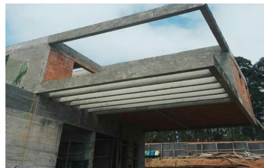
Fig.2 Real structure of cantilever by structville
