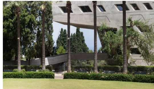
Fig.20: cantilever arm of 21m long floating above an open courtyard of double height Photographed by: Luke Hayes
