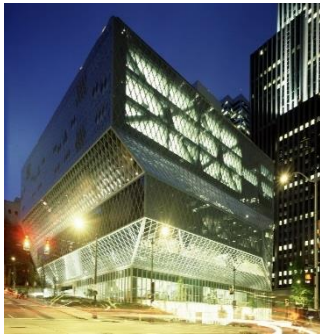
Fig.16: Real picture of library by archdaily
