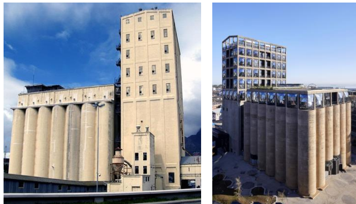
Fig. 4: The Grain Silo Before and After
